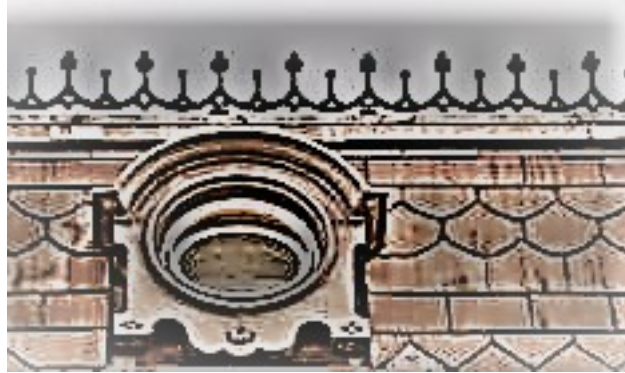
Example of an ornamental iron roof balustrade.
