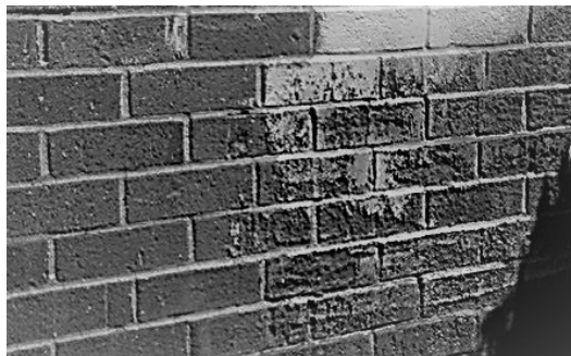
Effects of sandblasting on brick surfaces.
